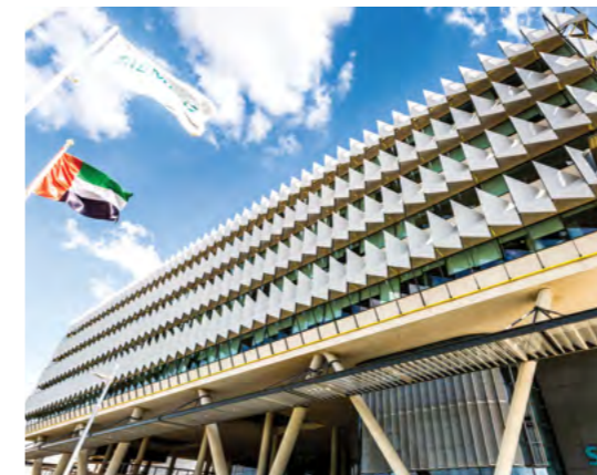
Siemens Middle East HQ at Masdar City
