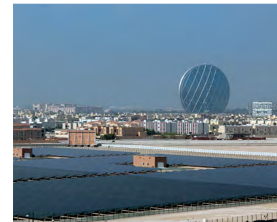
The Solar PV Plant at Masdar City
