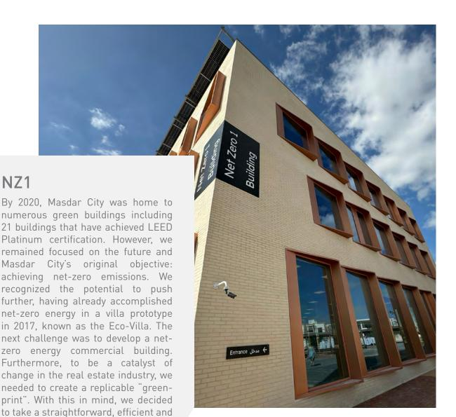
Drawing on over a decade of sustainable development expertise, we integrated lessons learned—such as advanced air-tight building envelopes, high-performance insulation, optimized window-to-façade ratios, and strategic solar shading and orientation. Our approach resulted in an impressive 53 percent reduction in energy demand compared to standard benchmarks, marking it as Masdar City's most energy-efficient building to date.
