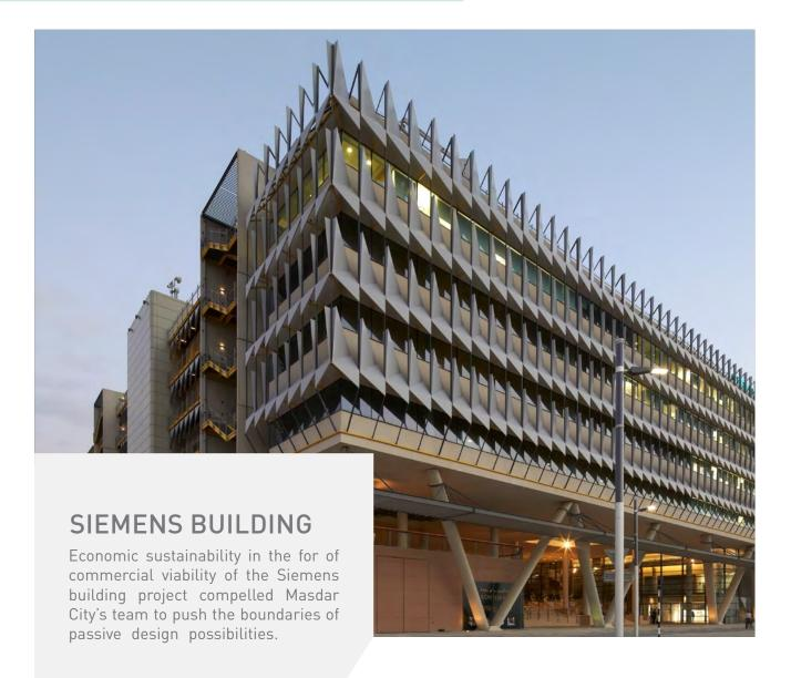
The Siemens Building is compact in form, being practically square on plan. Compact buildings can lead to less façade area which, in the case of Masdar City, reduces heat transfer from the exterior to the interior of the building. This approach to passive design also has cost benefits since less façade area requires less quantities of construction material to complete the building envelope.
